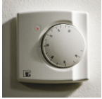
Wall-mounted room thermostat
